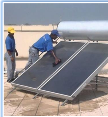
Solar Water Heater Repairing
